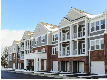
NORTHGATE CROSSING WHEELING, IL 288 UNITS
