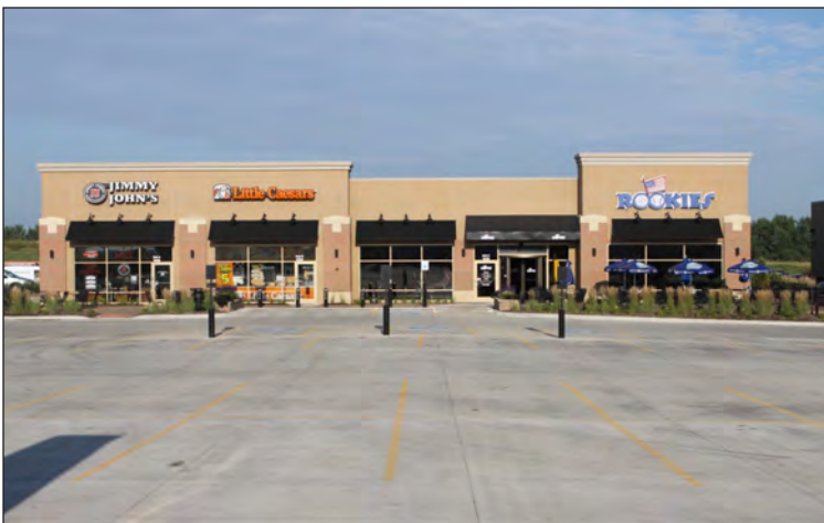
Parking lots and drives are concrete.
